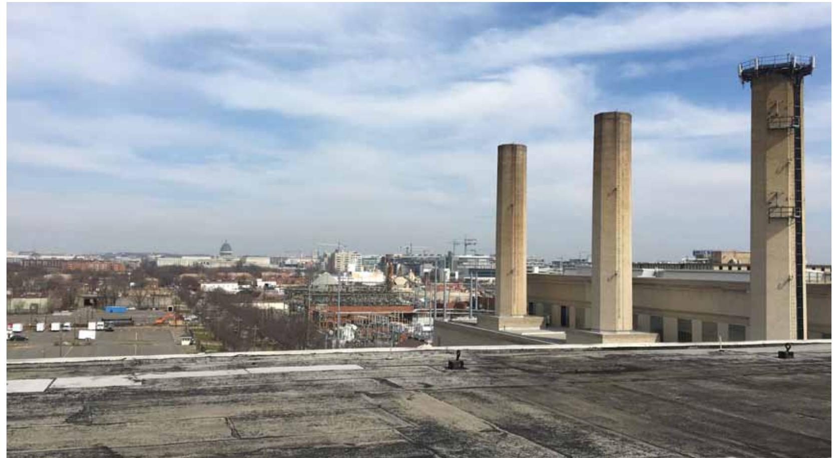
2. VIEW FROM NORTHEAST CORNER
