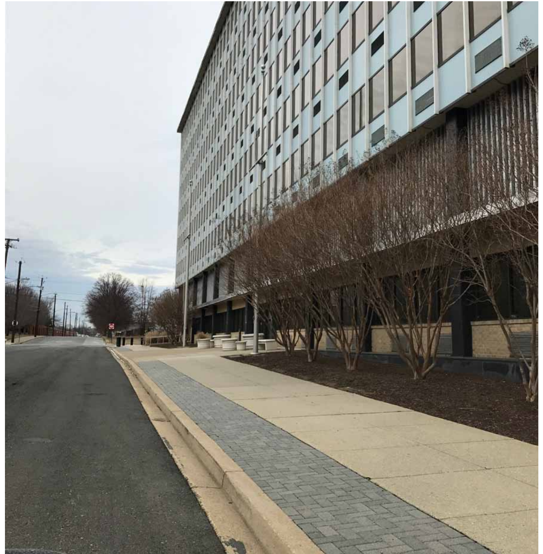
4. LOOKING NORTH ON 2ND ST, SW
